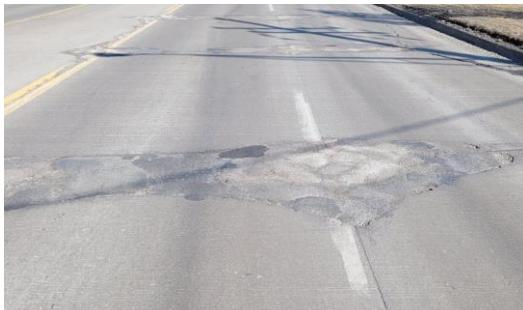
This project includes concrete repairs of deteriorated concrete pavement between 14 Mile Road and Metropolitan Parkway. The project will extend the roadway life and mitigate the need for the cold patches that have been used extensively this winter due to the freeze/thaw cycles and winter wear.
